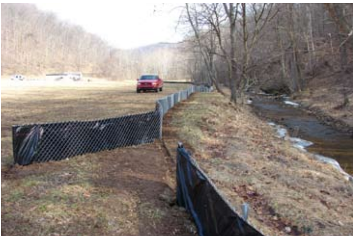
FIGURES II-7 Sediment Barrier Examples
