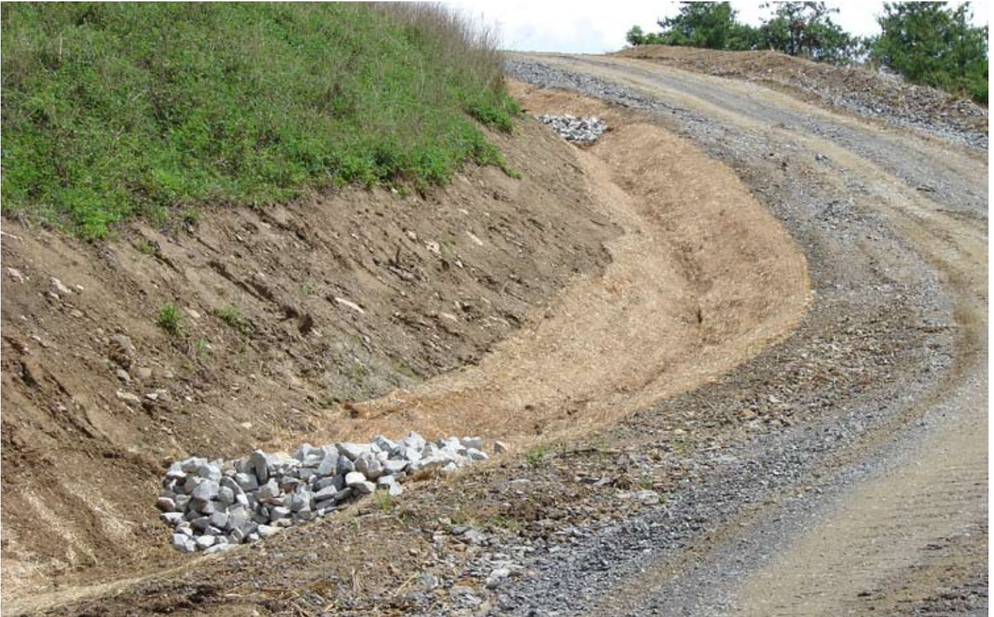
FIGURE II-5 Rock Ditch Check Dams
