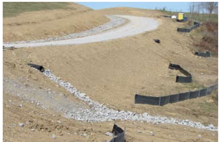
FIGURES II-7 Sediment Barrier Examples
