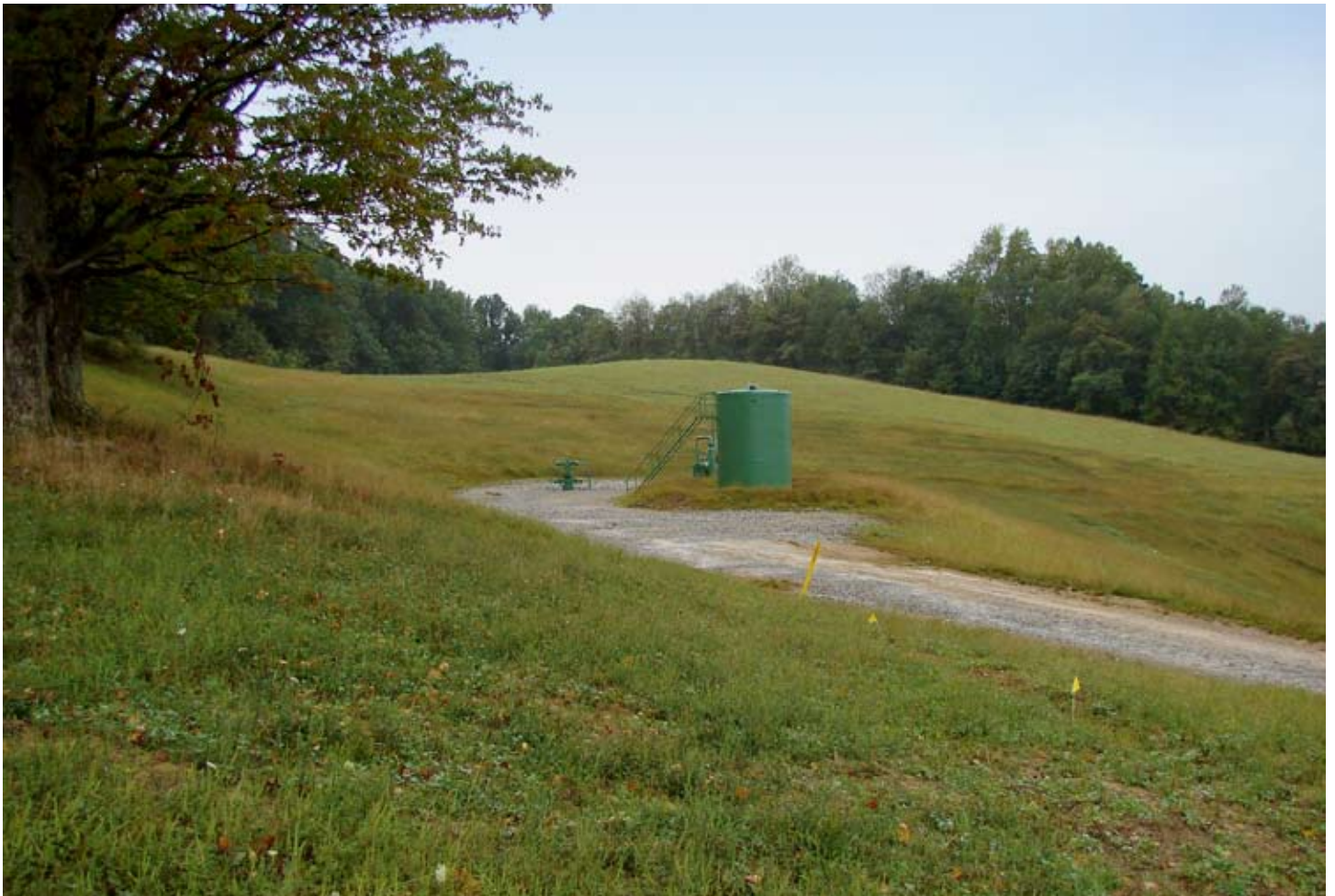
Example: Reclaimed Shallow Well Site
